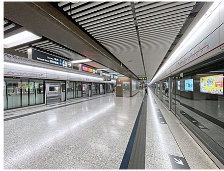
Platform screen doors installed at Central station on the Tsuen Wan line
